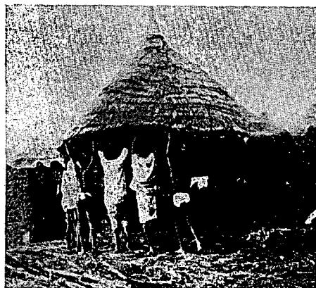
Raising the roof
